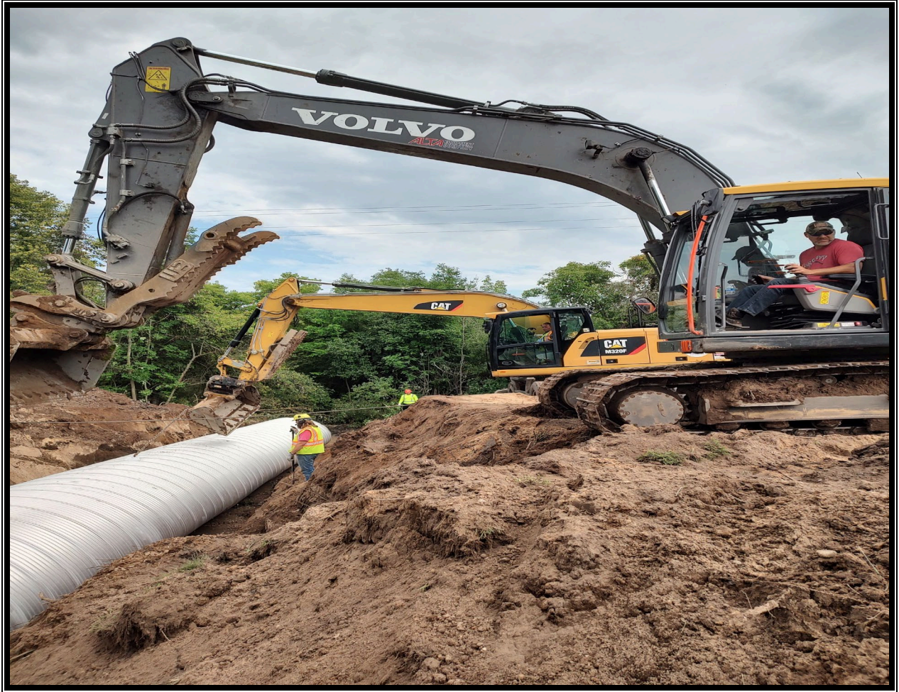
Culvert Replacement on Hawley Road
