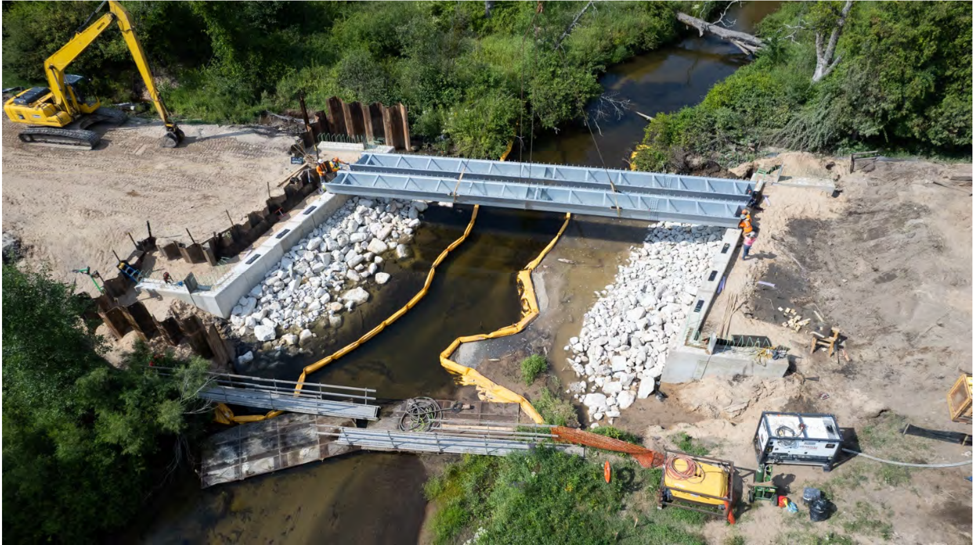
Setting Bridge Beams on concrete abutment walls - heavy rip-rap placed for scour protection
