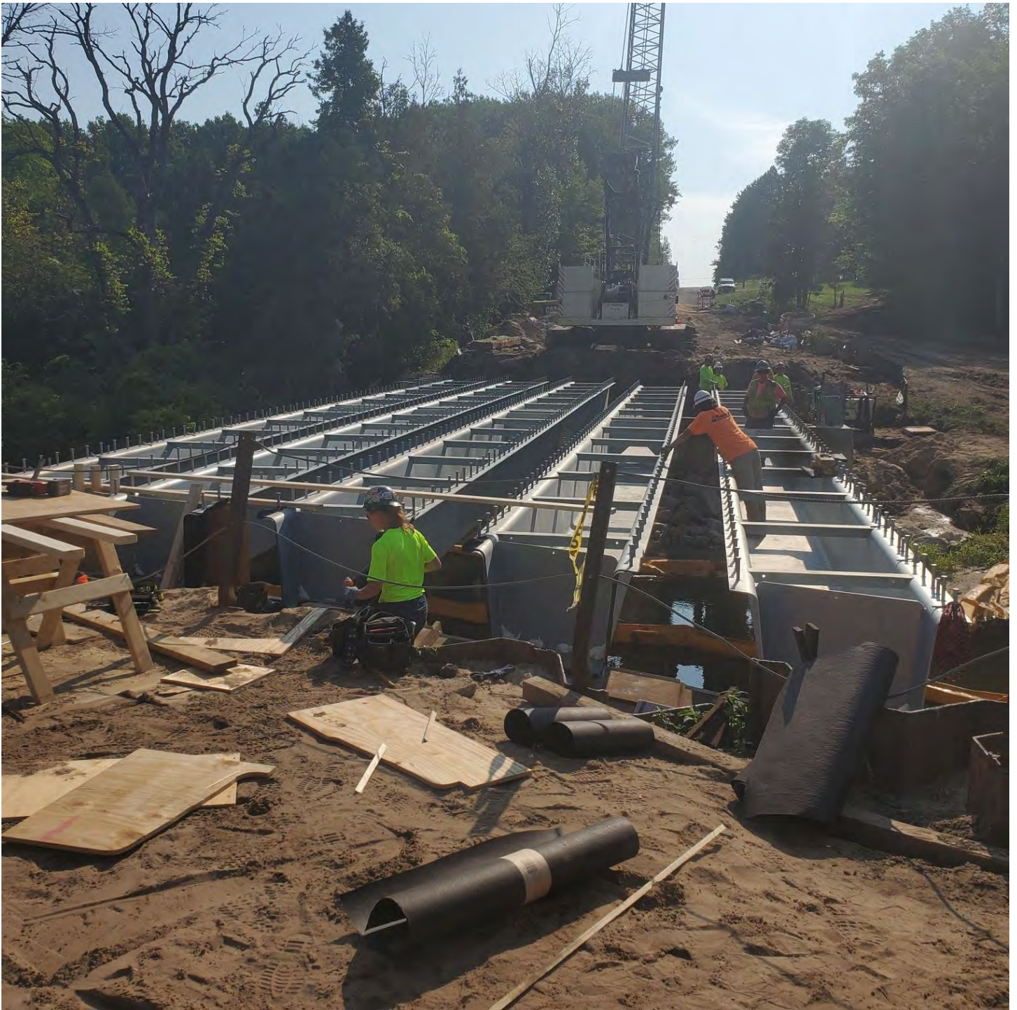
Five tub girder bridge beams set on concrete abutment walls
