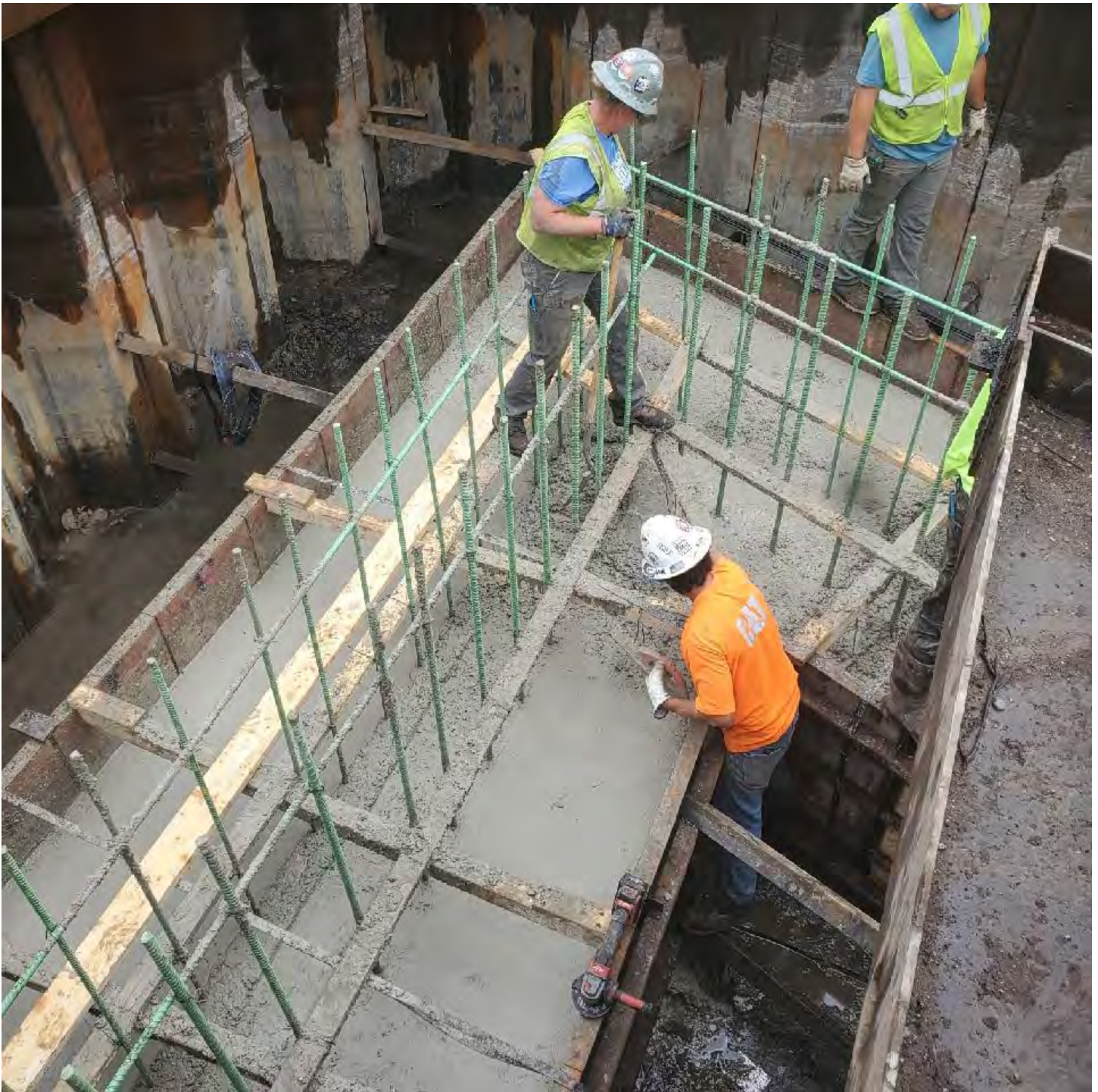
Pouring Concrete Footings over the steel piles
