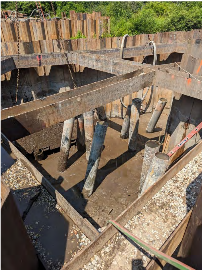
Support piles driven 60'+ deep to support the concrete footings
