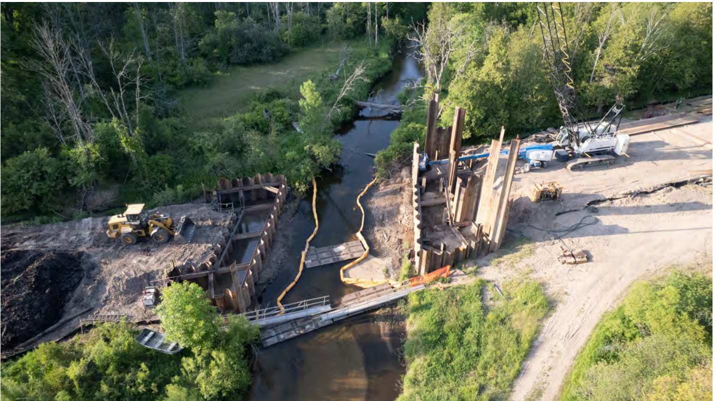
Installing Steel Sheet Pile Cofferdams - June 2023
