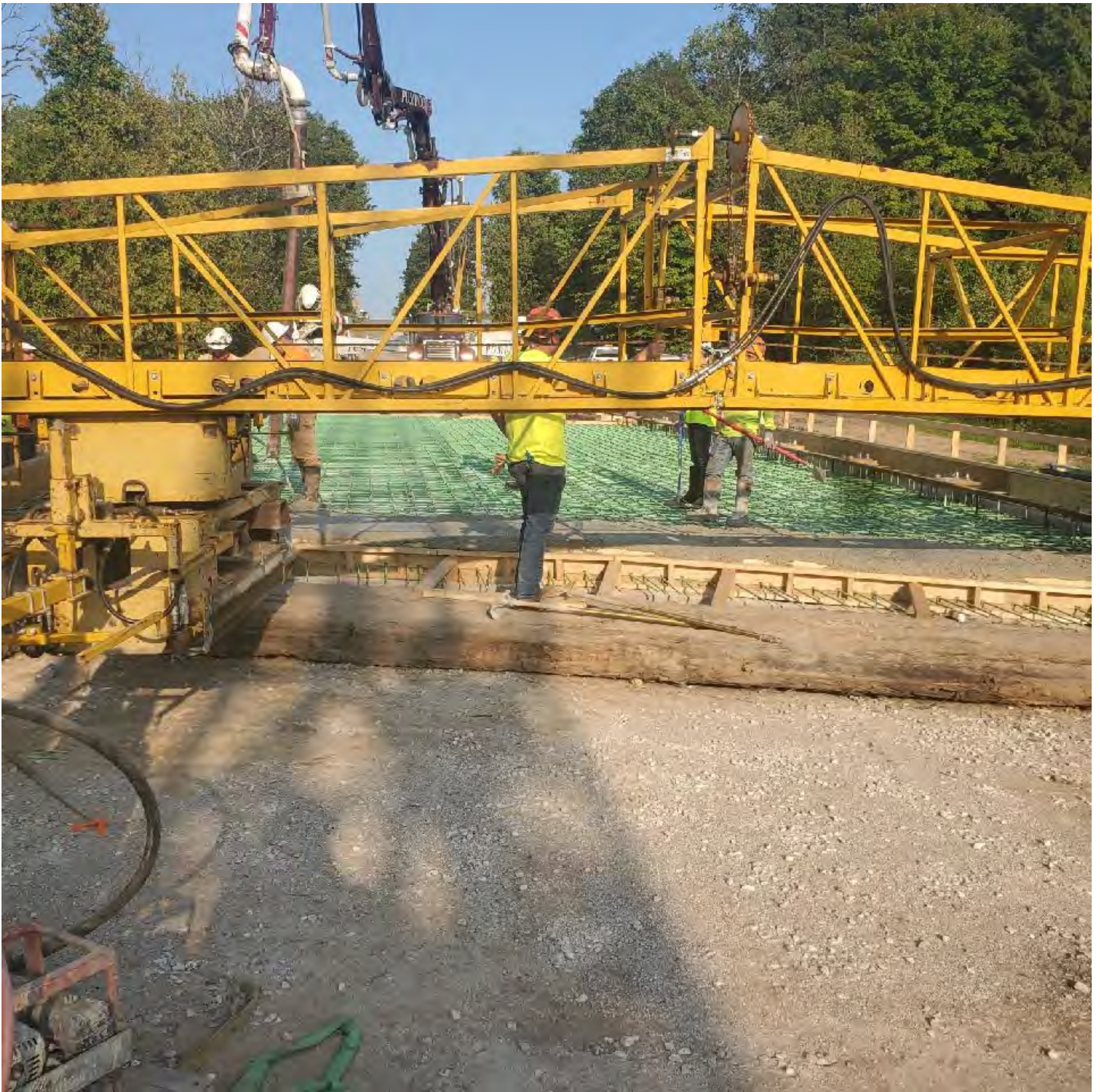
Pouring Concrete Deck - August 18, 2023
