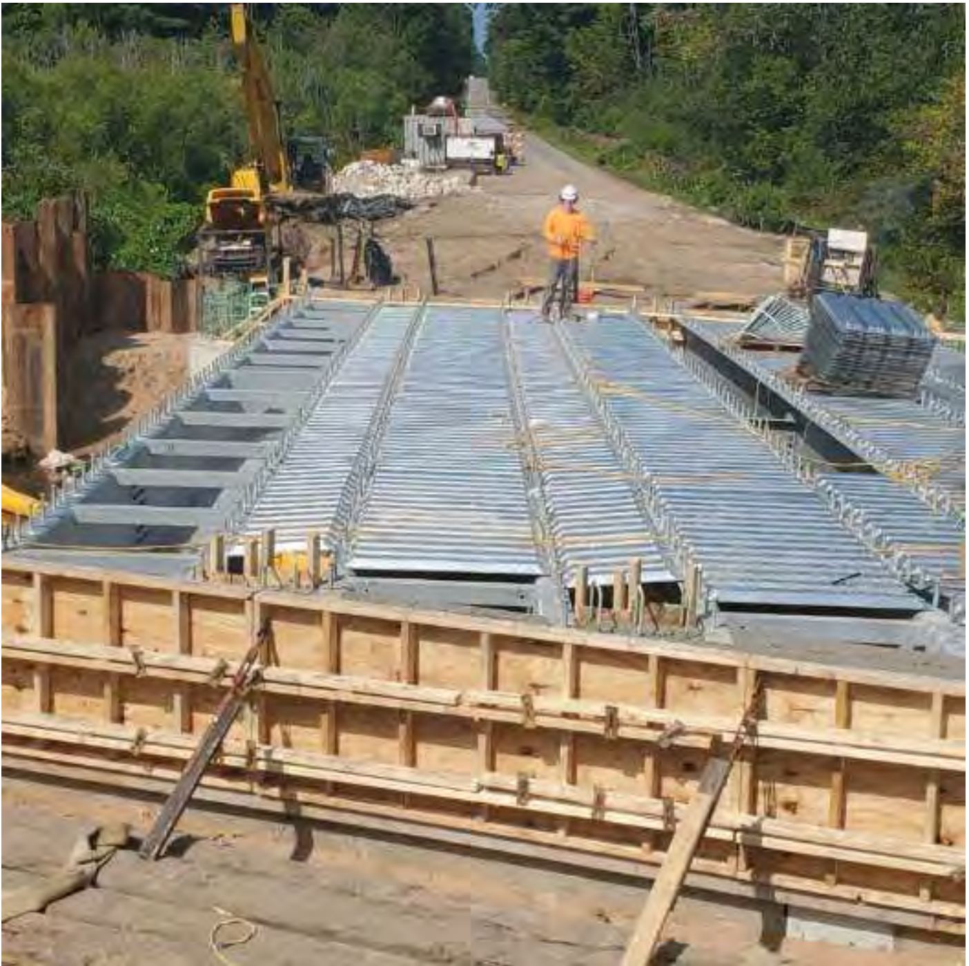
Pan Decking Installed on top of Tub Girders - August 2023
