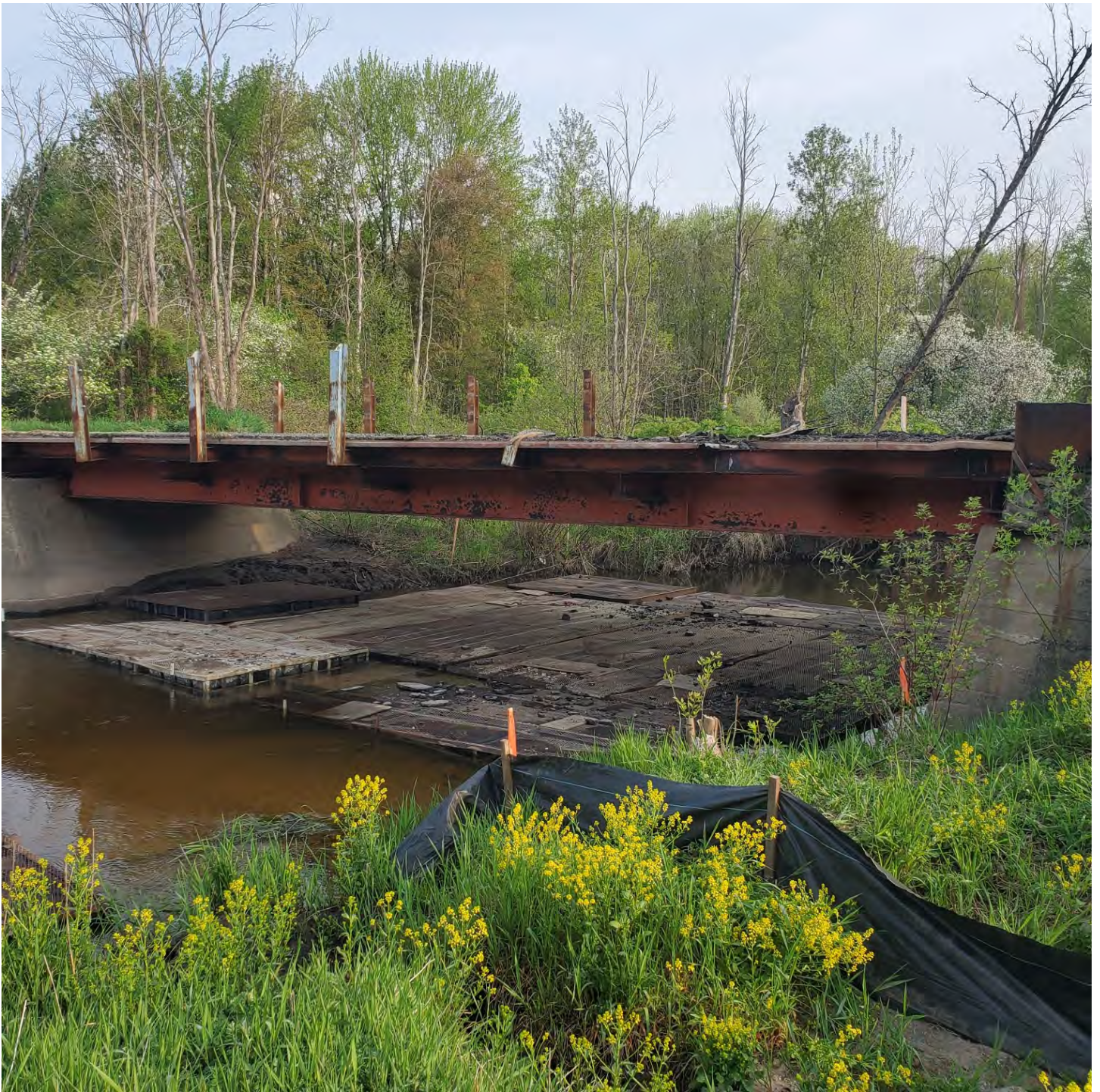
False Decking below bridge to catch any debris from falling into the Lincoln River
