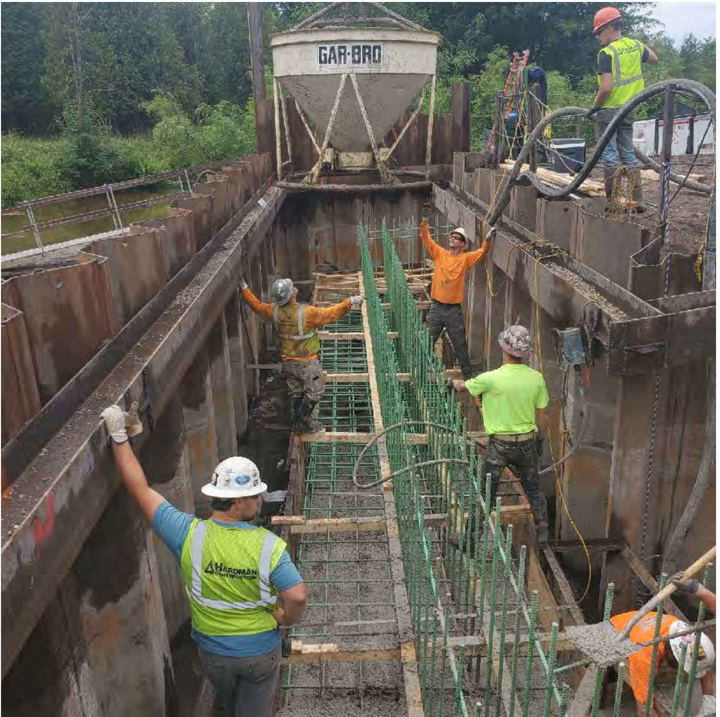
Pouring the concrete footings - July 2023
