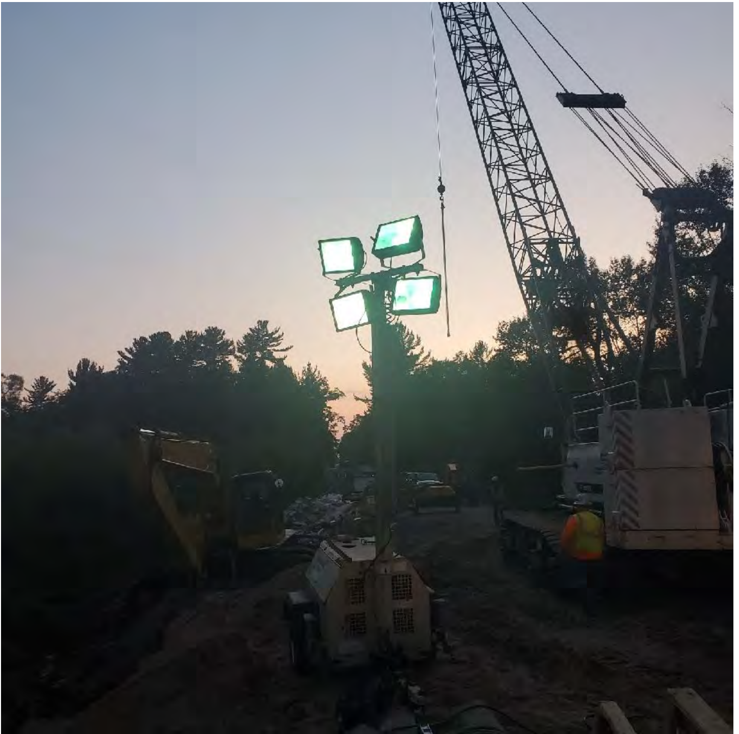
Light plants used for finishing the concrete deck after sunset
