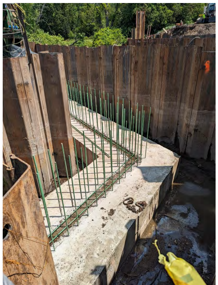
Support piles driven 60'+ deep to support the concrete footings
