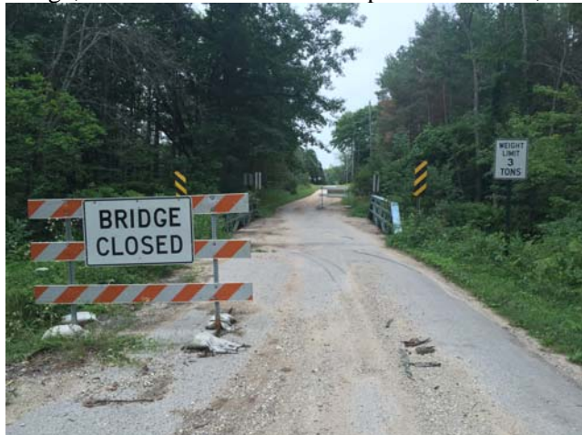
Figure 2 – View from approach
