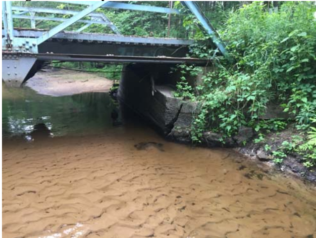
Figure 3 – View of abutment
